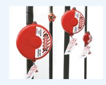
**In all Lockout procedures** an employee or maintenance team doing the servicing must have exclusive control of the lockout devices and padlocks.
